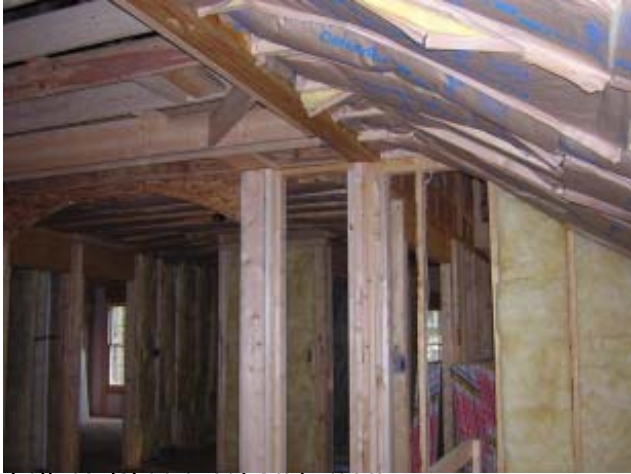
Loft insulation over Family room
