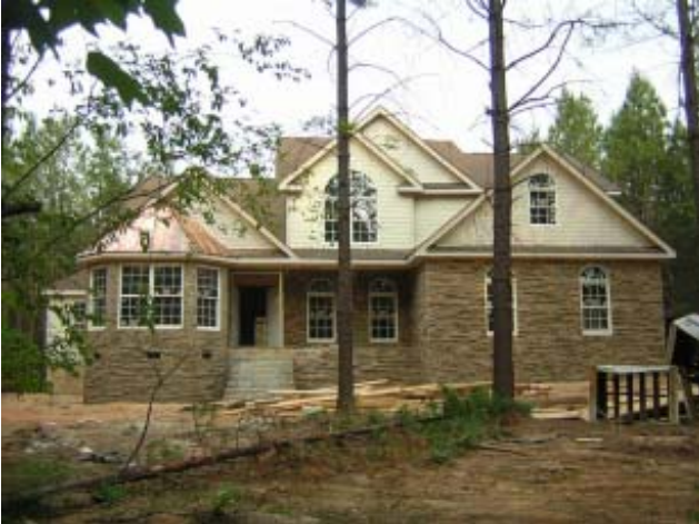
Frt elevation, copper roof,stones & Shake siding.
