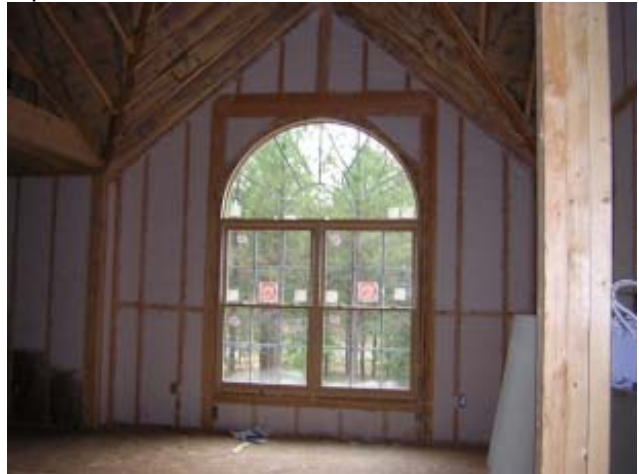
Master BR2 Spider insulation.
