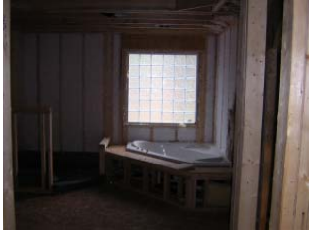
Spider insulation in Master Bath2
