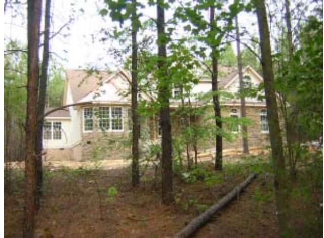
Frt elevation, copper roof,stones & Hardie K room.
